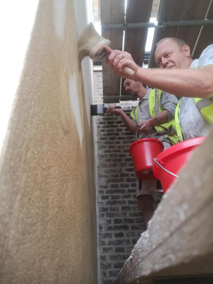
Decorators applying KEIM Restauro Lasur over KEIM Soldalit.
